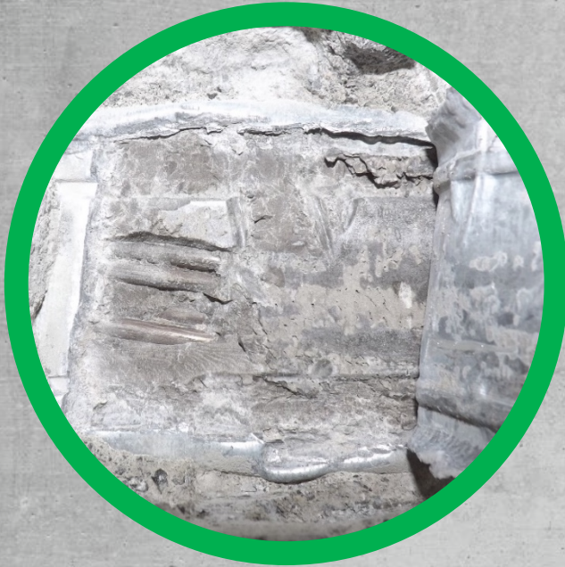
Properly Grouted No Corrosion
